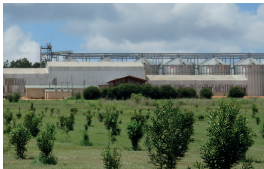
Silo complex and feed mill, Silverlands Tanzania
