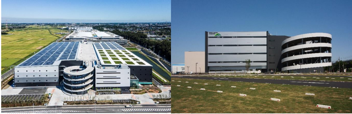
L: GLP ALFALINK Nagareyama, a LEED Gold certified logistics campus R: GLP Misato III, the first LEED Platinum certified logistics facility in Japan
