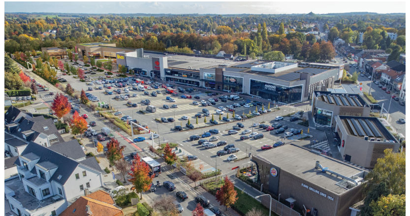
Sustainable Retail Park Waterloo, Belgium
