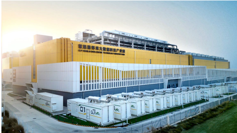
GLP Huailai Data Center, Hebei Province
