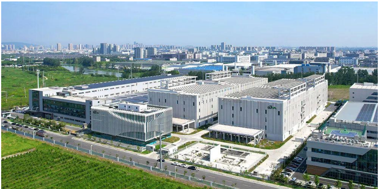
GLP Changshu Southeast Data Center Phase II
