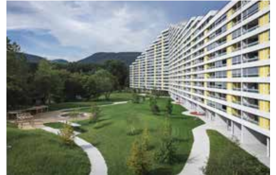
Prefabrication, modular construction, and lean management minimized renovation time at Telli Areal, Switzerland. © Sophie Stieger
