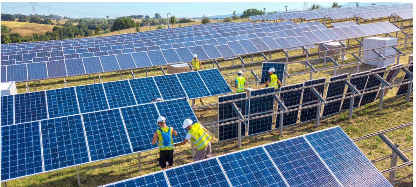
In a solar park in Italy, a KGAL asset manager discovered flaws in the solar modules at an early stage that would have led to a failure in the medium term. KGAL asserted the warranty claim in lengthy negotiations and replaced 73,000 solar modules worth around € 5.7 million at the manufacturer's expense.
