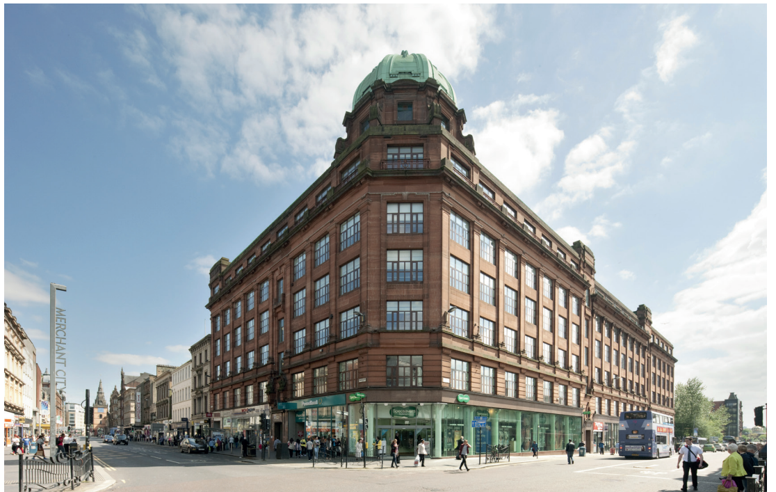
Granite House built in 1905, owned in partnership with Ambassador Group and funded by ICG, saw its energy efficiency improve threefold and achieved an EPC 'A' rating after a major refurbishment which helped reduce annual electricity costs by over 50%
